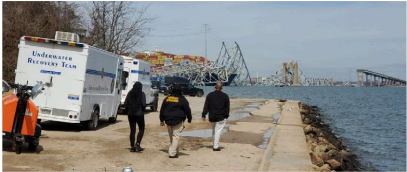
Baltimore City's Underwater Recovery Team truck with the collapsed bridge in the background
