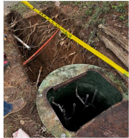
Major sewer project at the National Office
